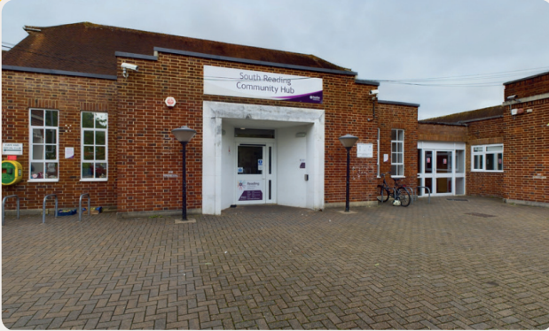
South Reading Family Hub 252 Northumberland Ave, Reading RG2 7QA 0118 937 3894
